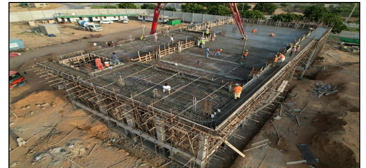
Construction of 132 kV Grid (Planned Completion in 2025)
